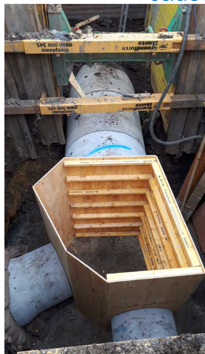
5) A trench is excavated where the metal sheets have been piled into the ground. The large pipes are installed in the trench. Manholes are constructed along at each change in direction of the pipework. The road is backfilled and reinstated.
