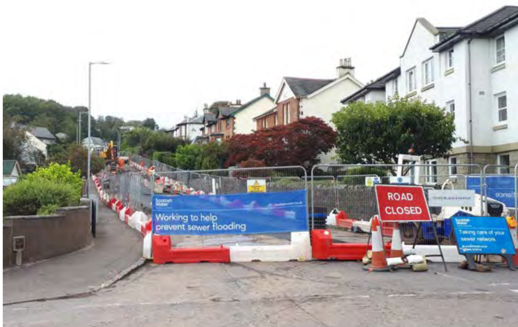
3) The working area of the road is fenced off .
