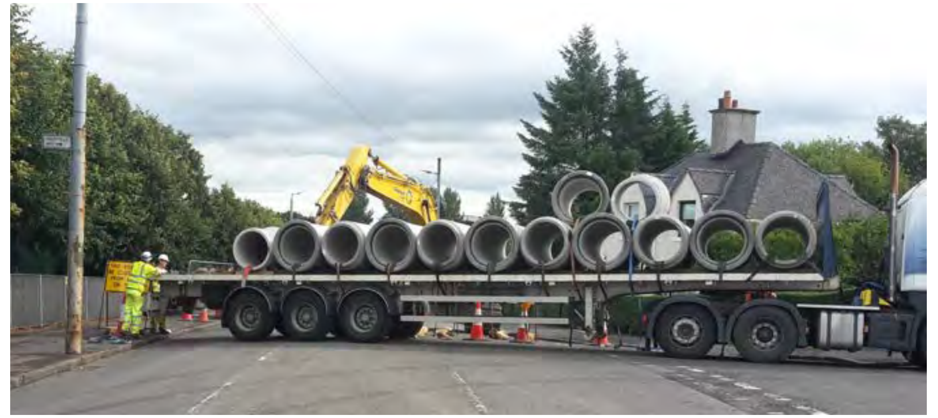
2) Large deliveries are made to site.
