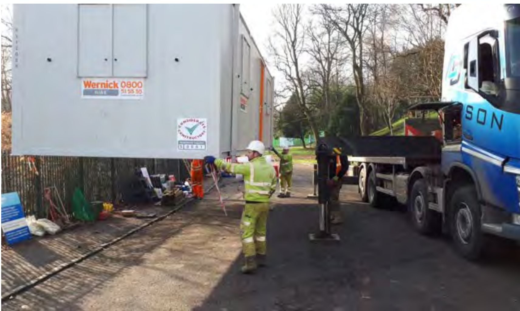
1) Site cabins are set up in the links.
