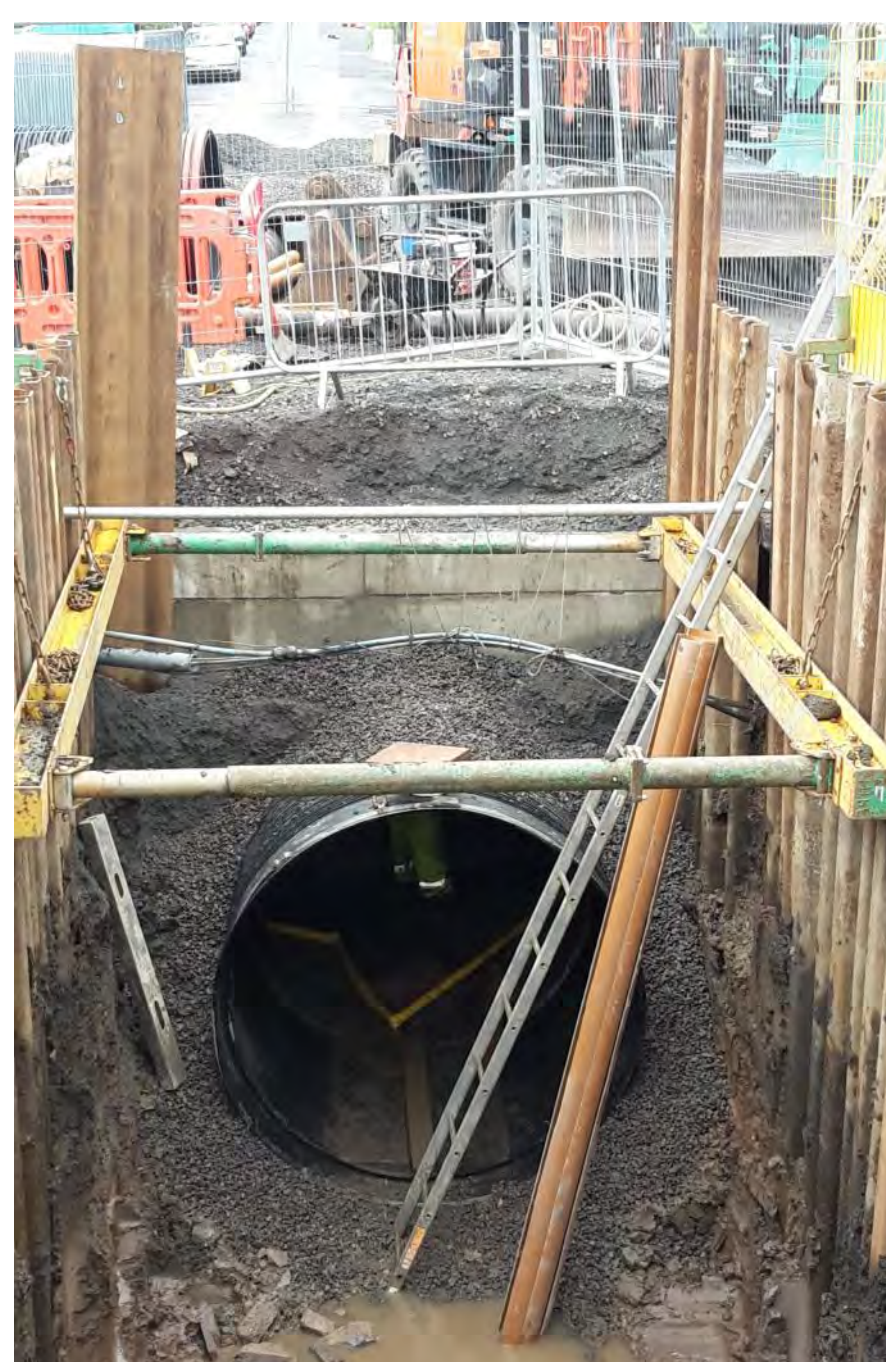
5) A trench is excavated where the metal sheets have been piled into the ground. The large pipes are installed in the trench. Manholes are constructed along at each change in direction of the pipework. The road is backfilled and reinstated.
