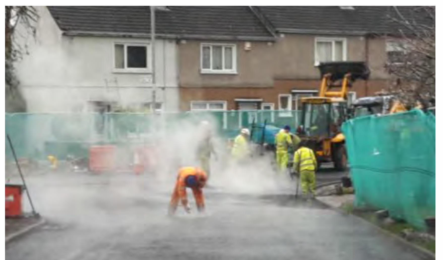
5) A trench is excavated where the metal sheets have been piled into the ground. The large pipes are installed in the trench. Manholes are constructed along at each change in direction of the pipework. The road is backfilled and reinstated.
