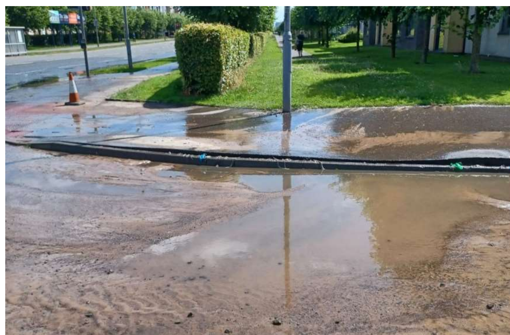
Burst incident on Kings Inch Road 2023
